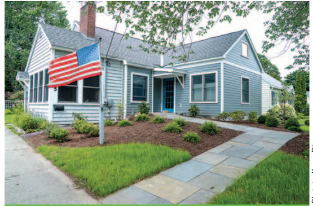
A "ramped" walkway replacing stairs
